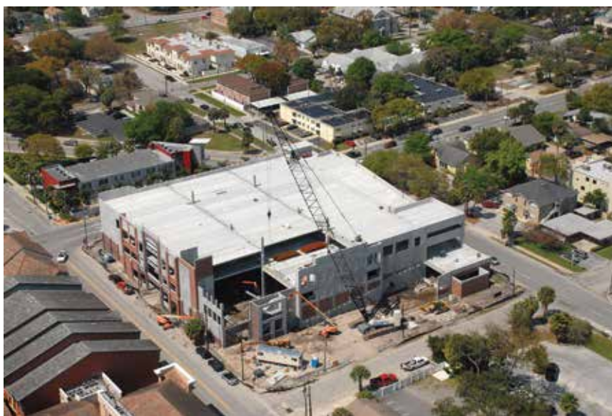
The Publix GreenWise in Tampa, Florida used architectural and structural precast in order to build the upscale, grocery store on a tight construction sight, as well as completed the project in about 2/3 the time as conventional construction. Top photo courtesy of Nino Giannotti. Bottom photo courtesy of Ariel Innovations, Inc.
